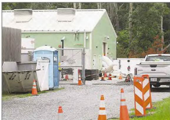
Lithium-ion battery storage facility substation at in East Hampton.
